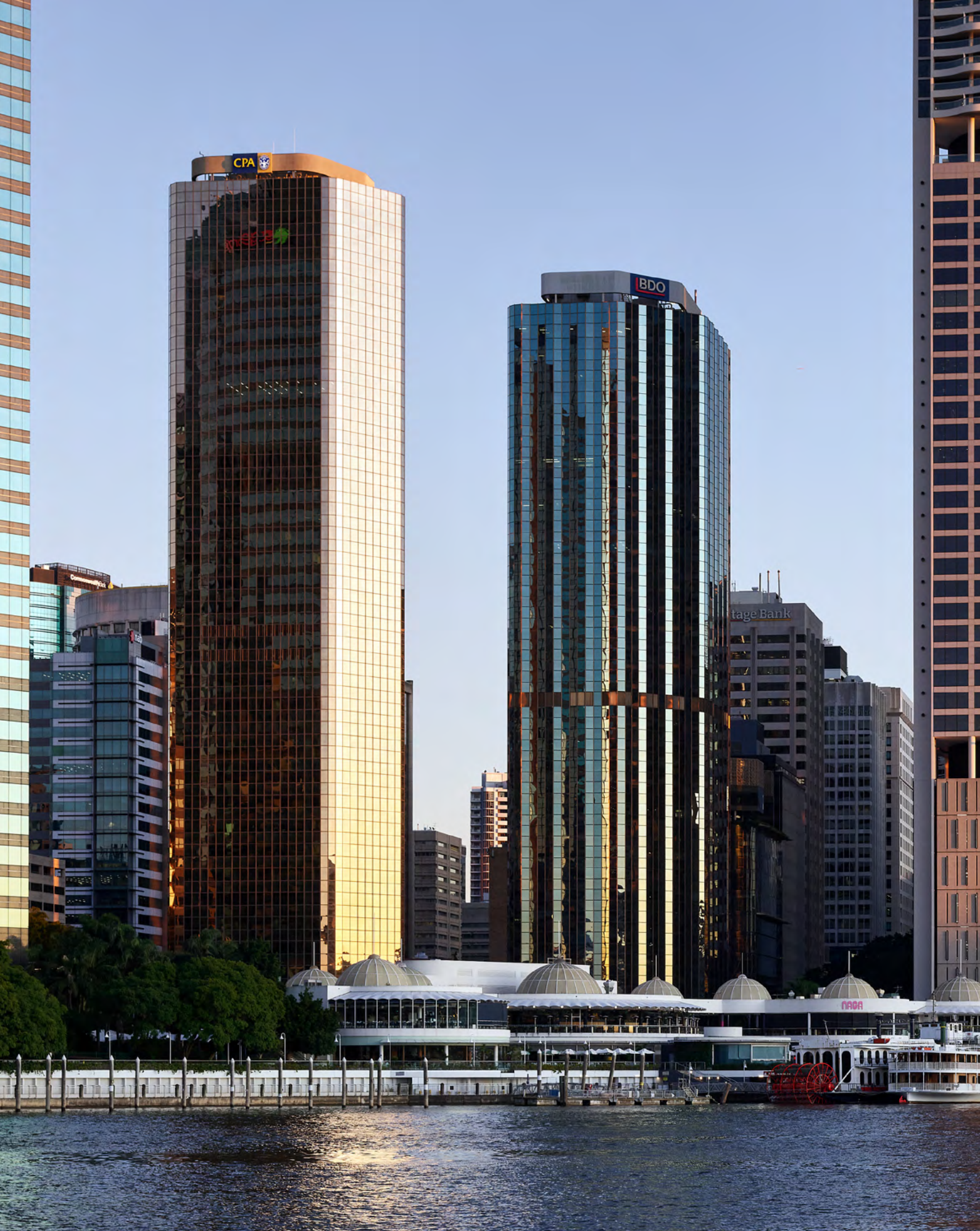
The Brisbane waterfront redevelopment site opposite Gold Tower and Blue Towers.
